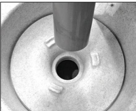
6. Refit the pipe assembly by pushing the shorter end back into the EazyPod, so that the long length is now the exit.
